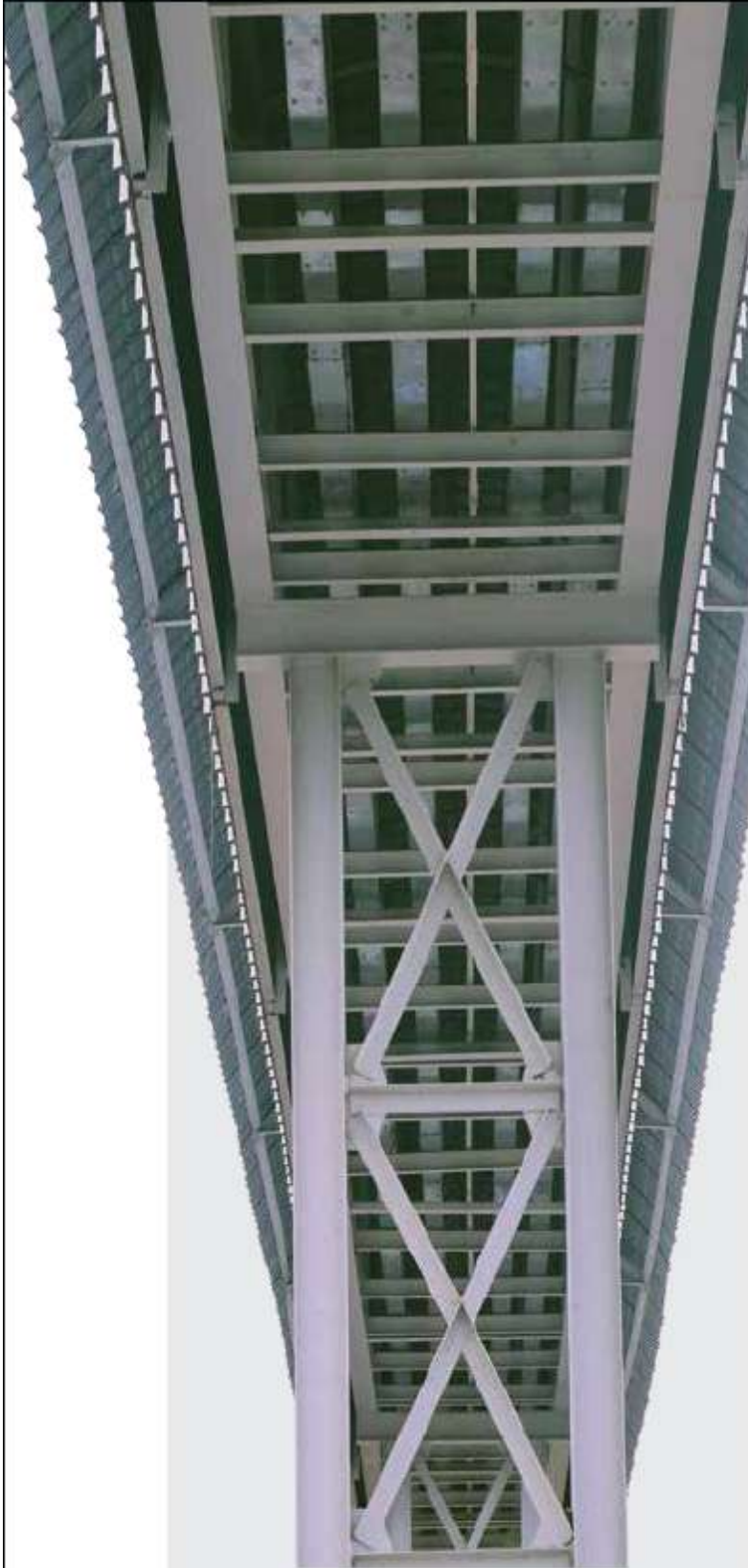
1.2 km Adex Busbar (BTA)
