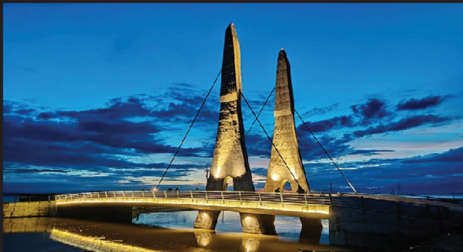
Bangabandhu Sheikh Mujib Hi-Tech Park, Sylhet
